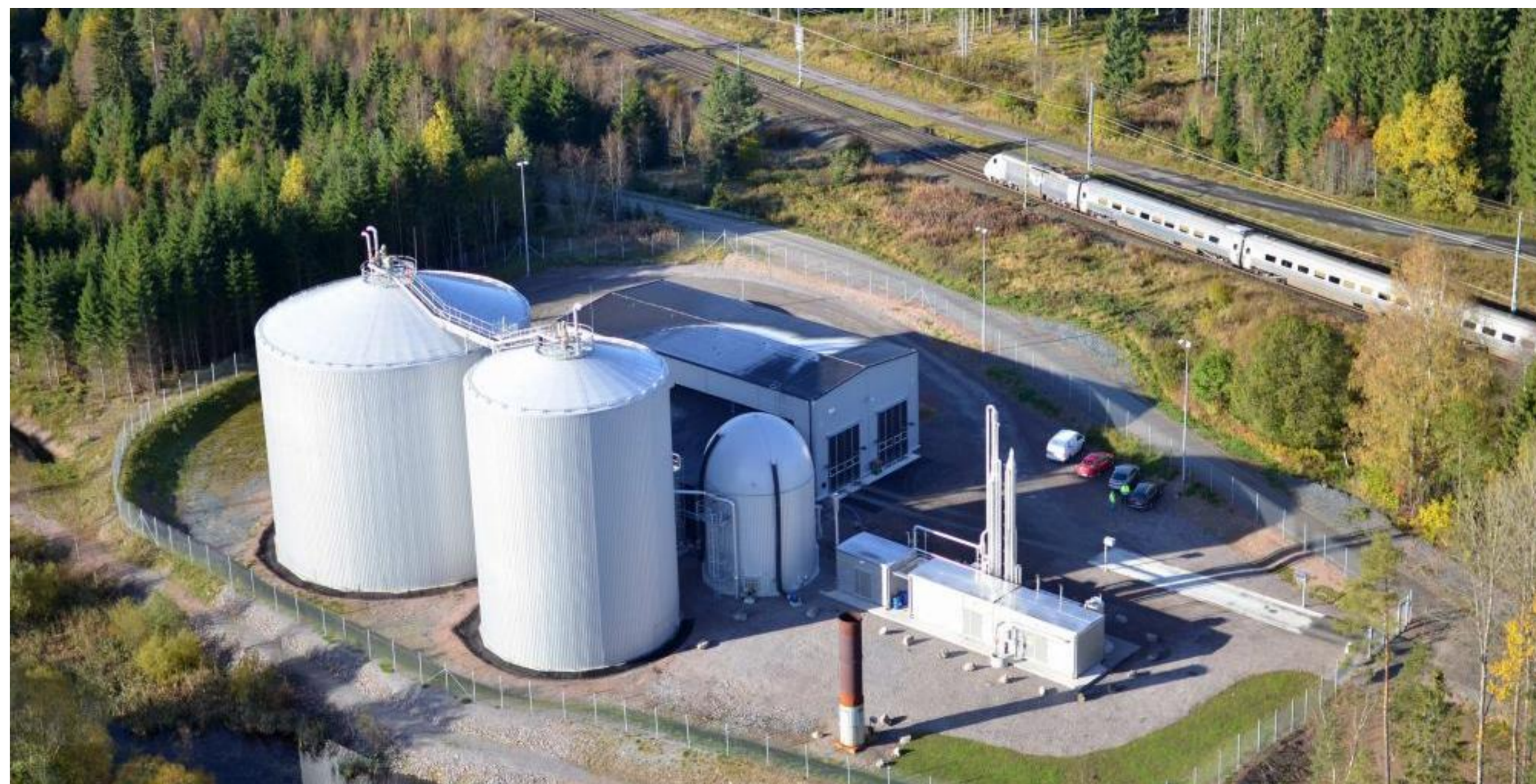
Figure 2: Thermophilic anaerobic digester (Sävsjö); source of inoculum and substrate for the present research.
